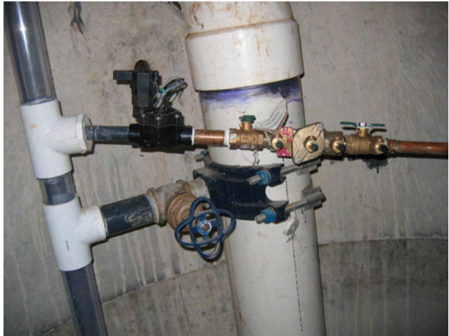
Auxiliary Water line with dual check valves and electric control valve
