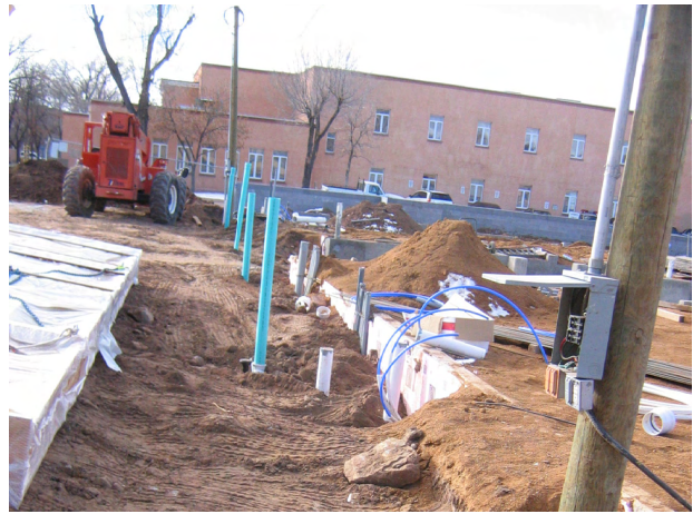
Roof Drops to Conveyance: January 2005
