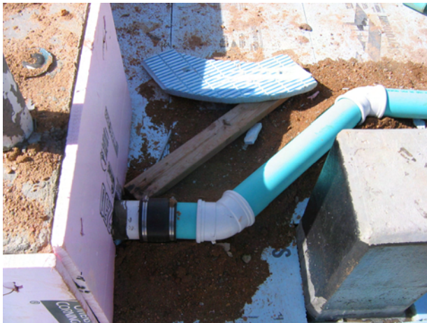
Roof Drop to Conveyance: January 2005
