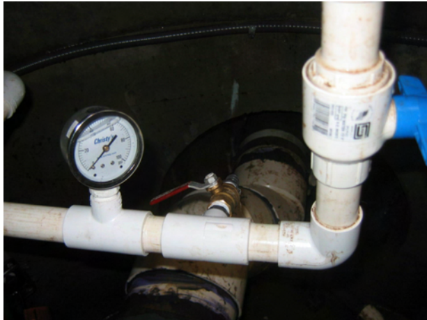
Irrigation Line Pressure Gauge and Line Flush Valve
