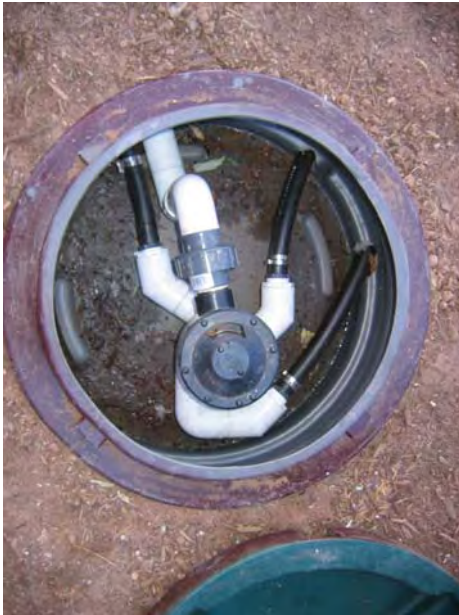
Mechanical Sequencer Valve. Distributes Greywater to three distribution lines
