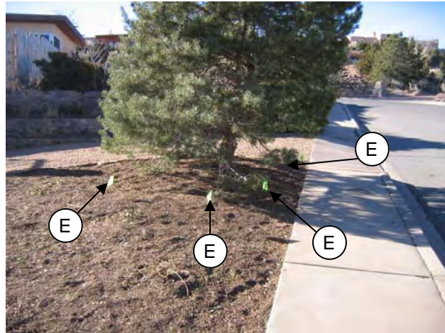
Greywater Zone 1 Emitters at Piñon and others at locust tree.
